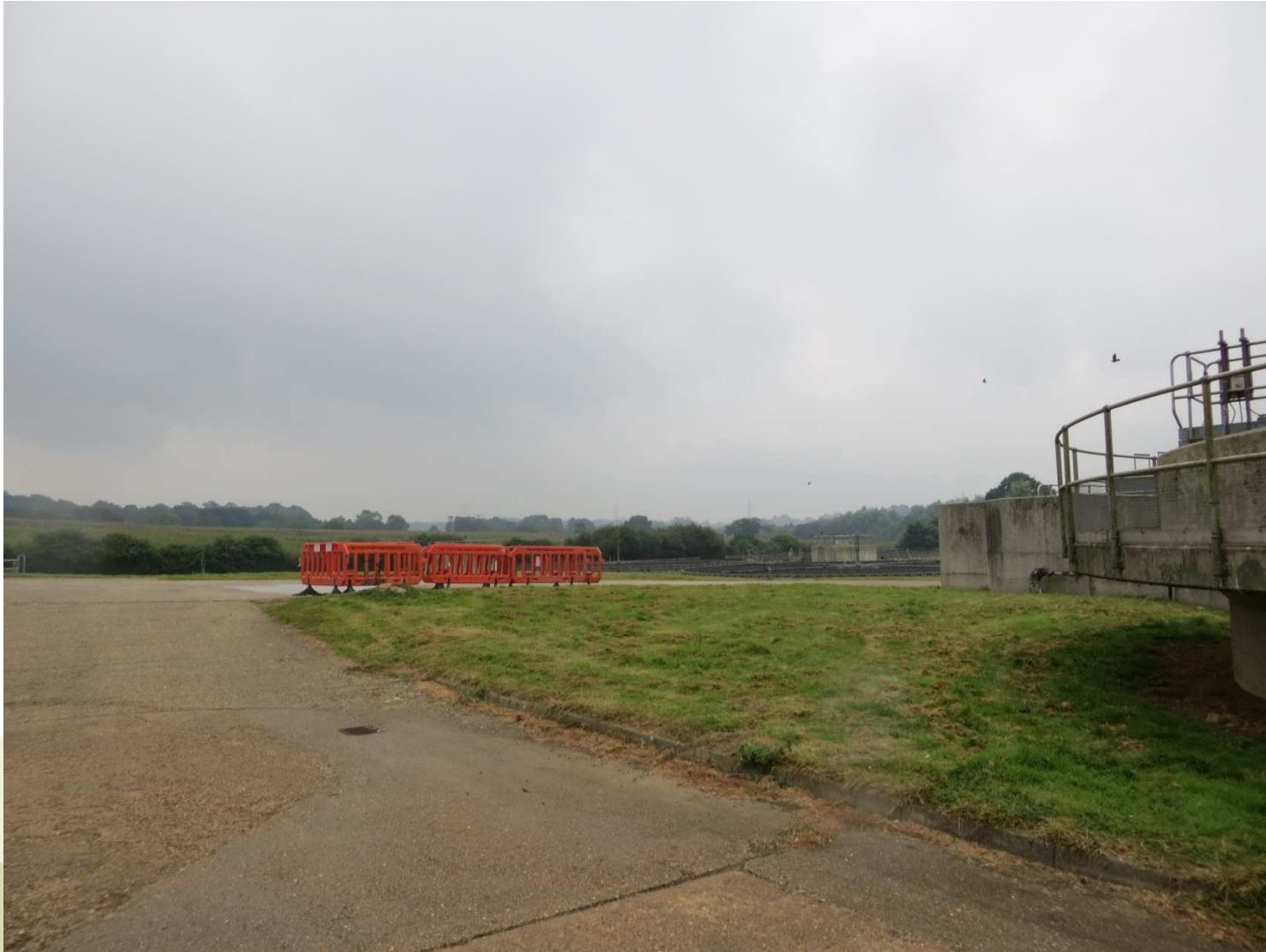
View looking south-west towards area of proposed Alkalinity Dosing Plant Kiosk
